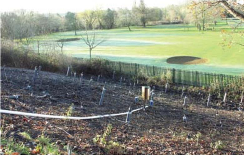
**Once the electrodes had been installed, the electro-kinetic remediation process took place over six weeks with no staff on site.**
