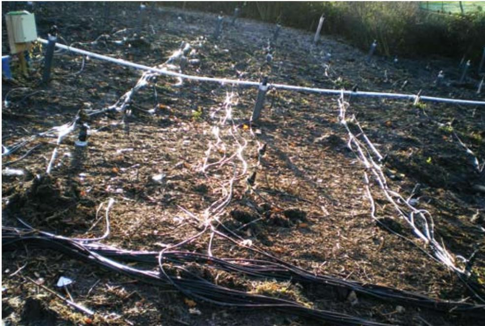
**SUPPORT** Trials in the UK have confirmed that electrokinetic geosynthetics can be used to stabilise embankment and cutting slopes, addressing underlying causes such as weak soils and poor drainage as well as providing physical reinforcement.
