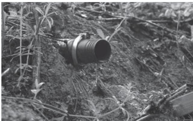
Figure 10. Cathode drain providing passive drainage at Stocks Green
