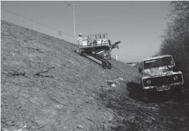
Figure 3. Small self-climbing rig for installation of EKG electrodes
